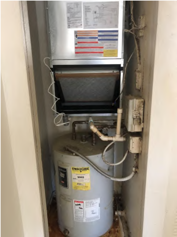
HVAC AIR HANDLER & WATER HEATER
